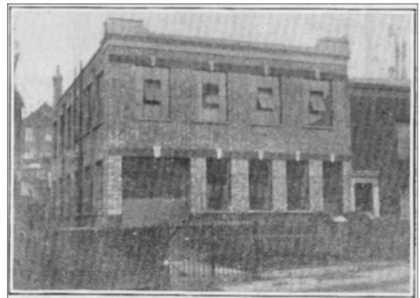
The New Printing Works Nearing Completion.
