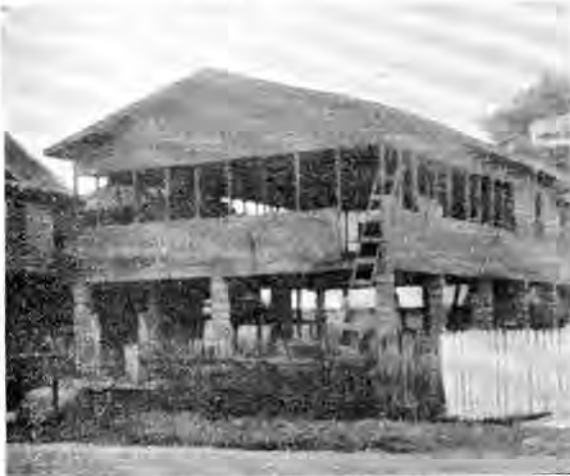
Church in construction, British Guiana.
