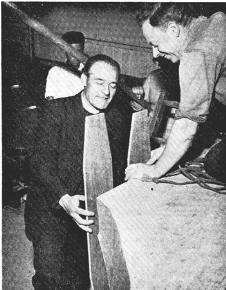
The platform being erected by Pastor Canty and church member.
