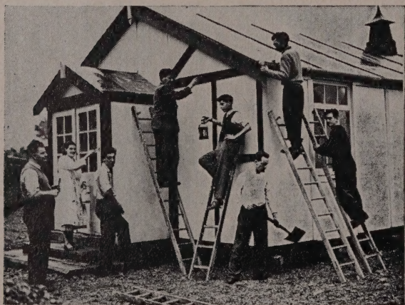
Members at work on Hadley's new church.
