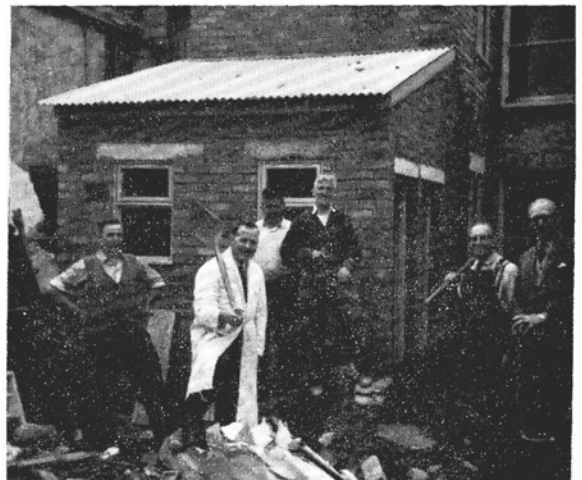
At work renovating the Neath manse.
