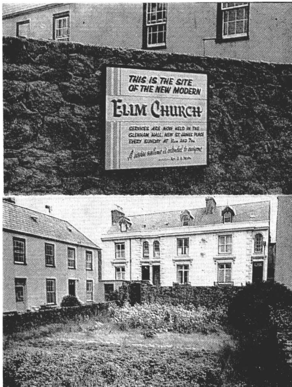
Views of the site of Jersey's new Elim church.
